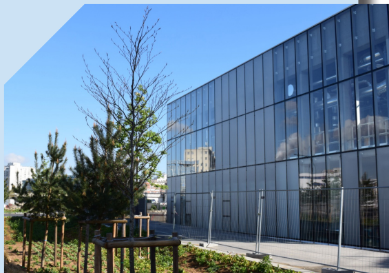
Centrale Géothermale Ivry Confluences photo © CPCU
