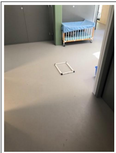
RDC - Circulation - Sol
