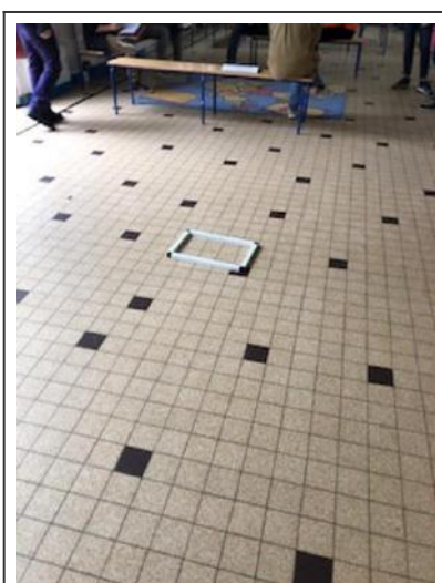
RDC - Hall - Sol
