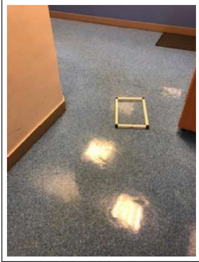
R+2 - Circulation - Sol
