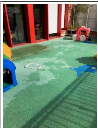
R+1 - Terrasse (petite section) - Sol
