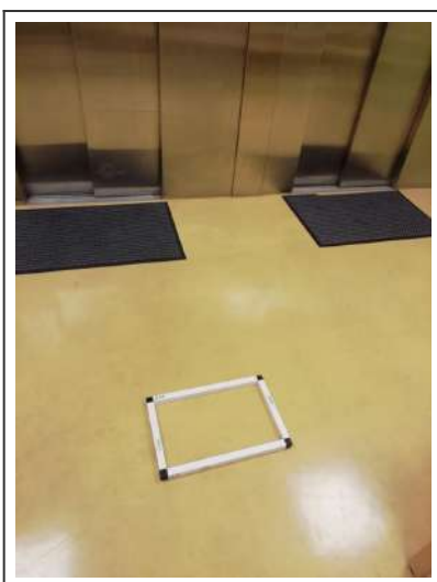
48 - R+3 - Hall - Sol
