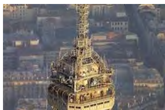
Emprises antennaires Tour Eiffel
