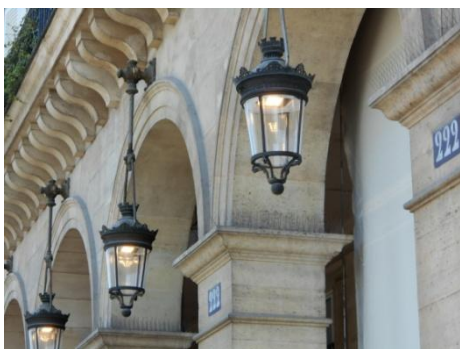
LED Lighting. © Paris City Hall
