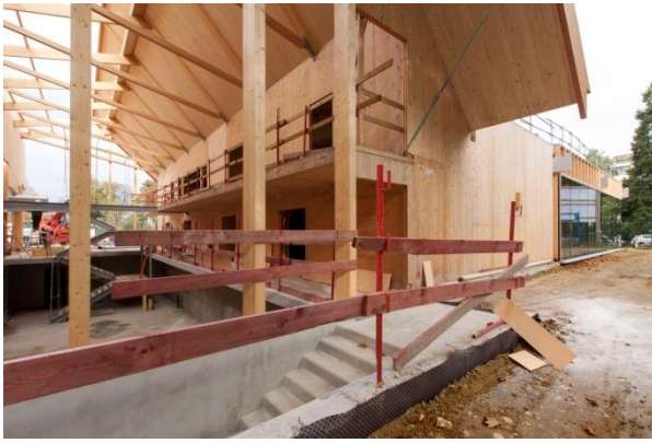
Wood construction of Suchet Gymnasium (16th) © Paris City Hall
