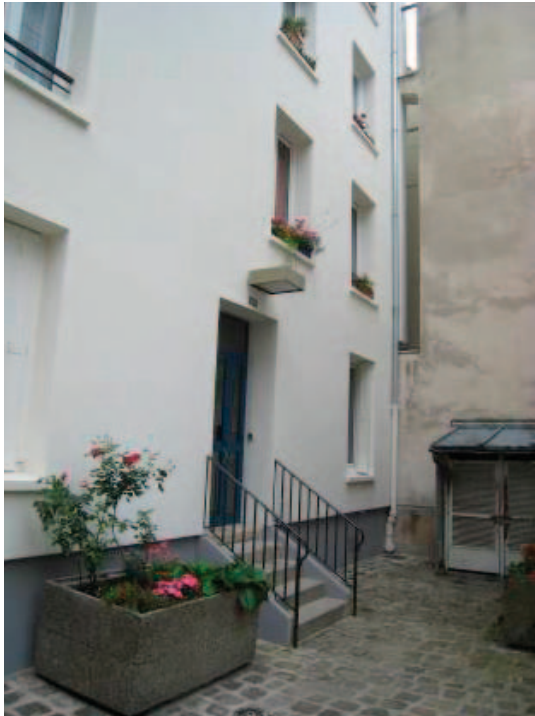
Building located on rue de la Roquette (11 th ) built at the beginning of 20th century – © Logement français
