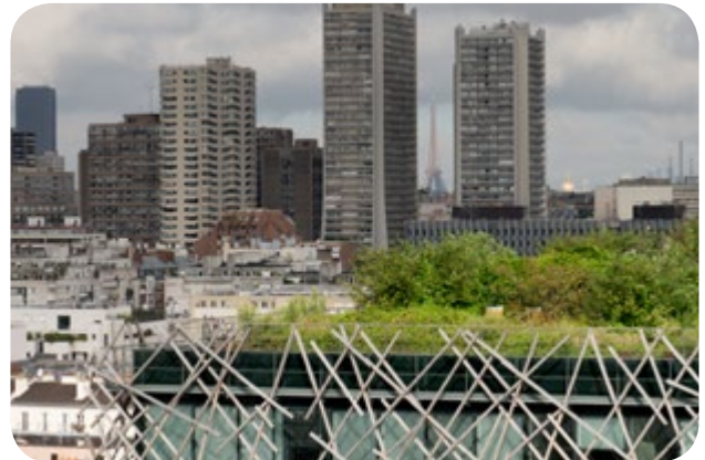
The roof of the administrative building 121 avenue de France (13 th arrondissement) is planted
