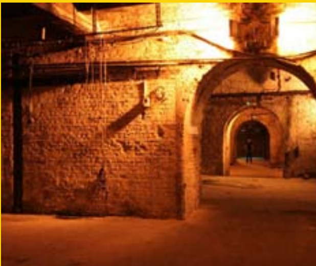
The Old Vic Tunnels (Source : www.lawfullychic.com)
