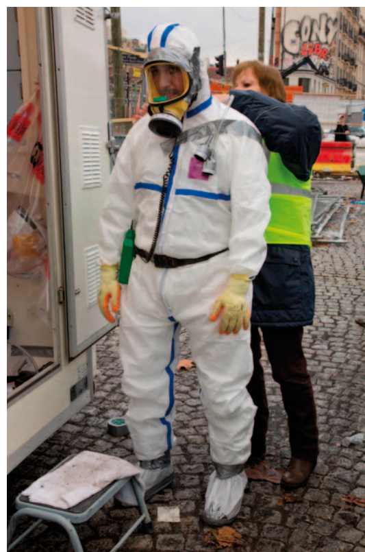
Hazmat suit for asbestos removal. © Mairie de Paris, DVD
