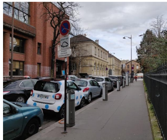
Station Mobilib' – rue Pierre Castagnou
