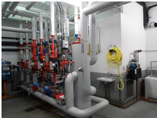
Example of a thermal center after renovation (Rue Poliveau 5 th arrondissement)
