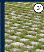
pavés joints sable
