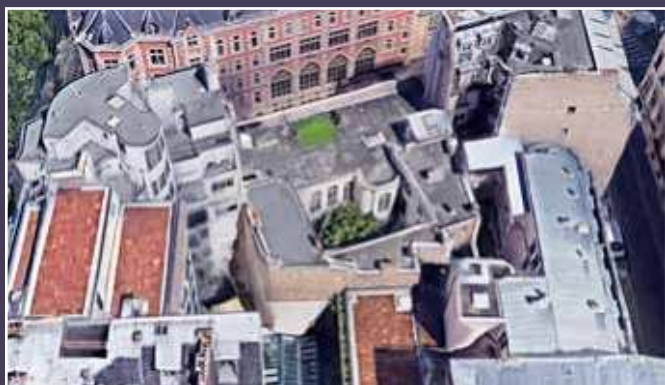
Current aerial view of the plot.
