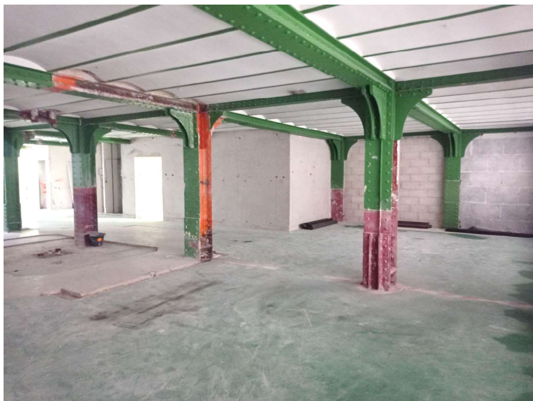
Curage © GIET architecture
