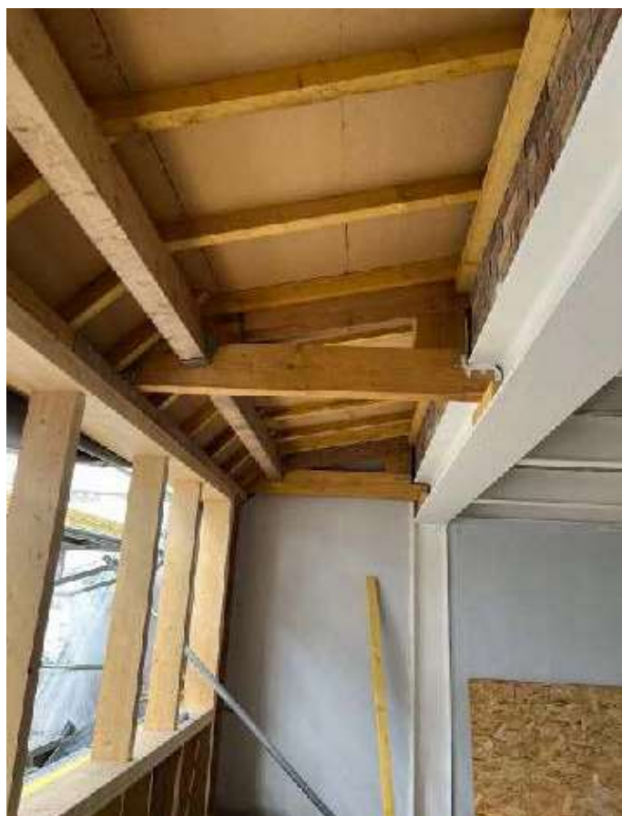
Enveloppe ossature bois © GIET architecture
