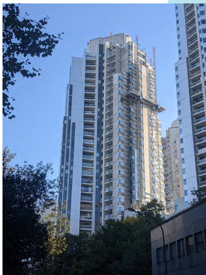
Tour Cantate, energy efficiency renovation worksite @Soliha
