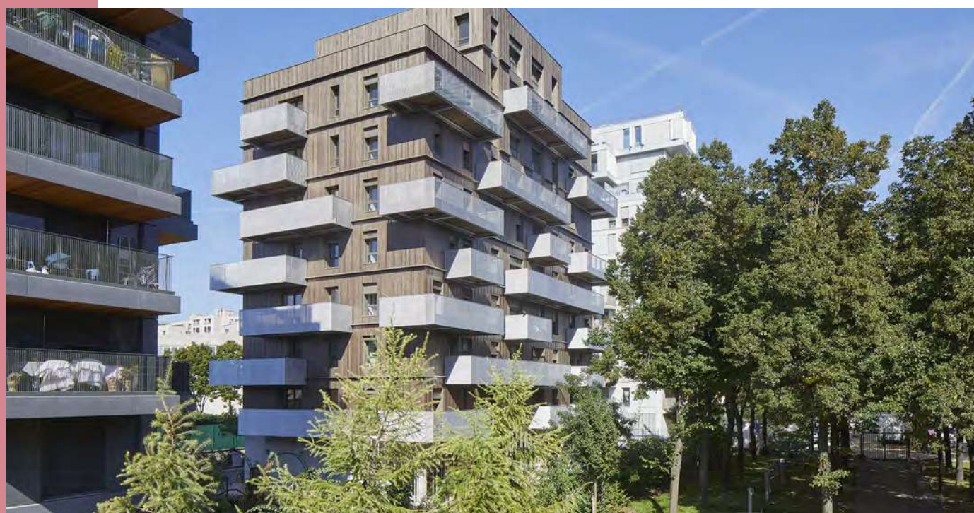
New construction, Paul Bourget, 13 th district @Hervé Abbadie
