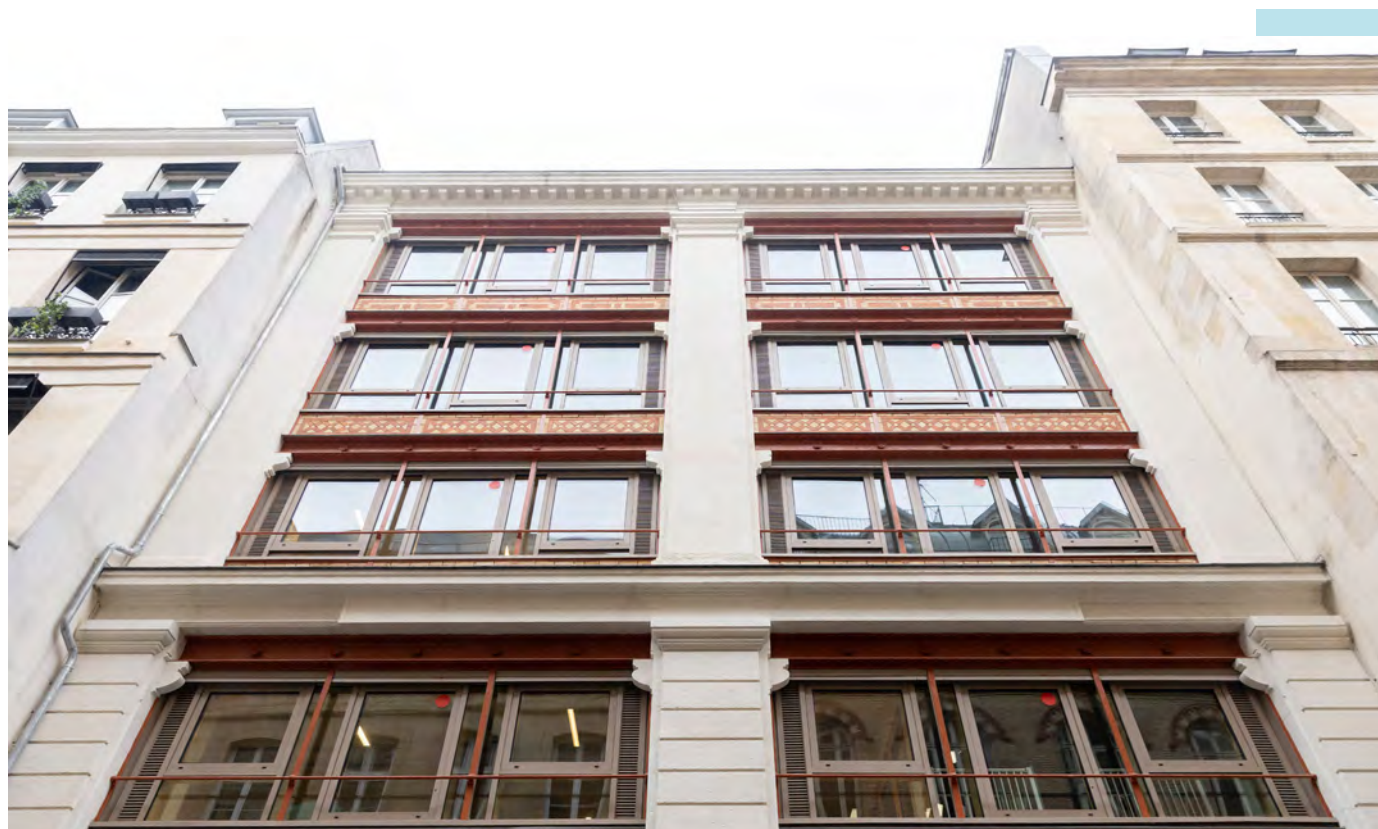
St Roch nursery façades after renovation @Joséphine Bruecker
